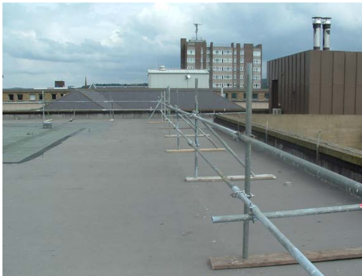
Temporary edge protection (scaffolding poles)
