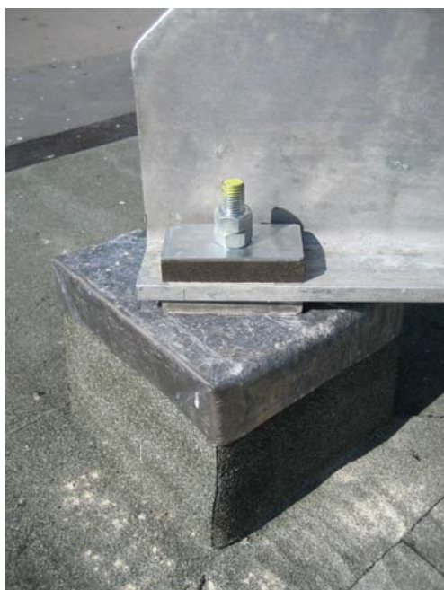
Mounting of wind turbine frame with vibration dampening pads
