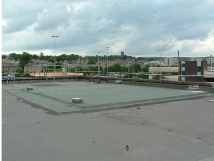
Thermal insulation prior to installation of wind turbine mounting frame
