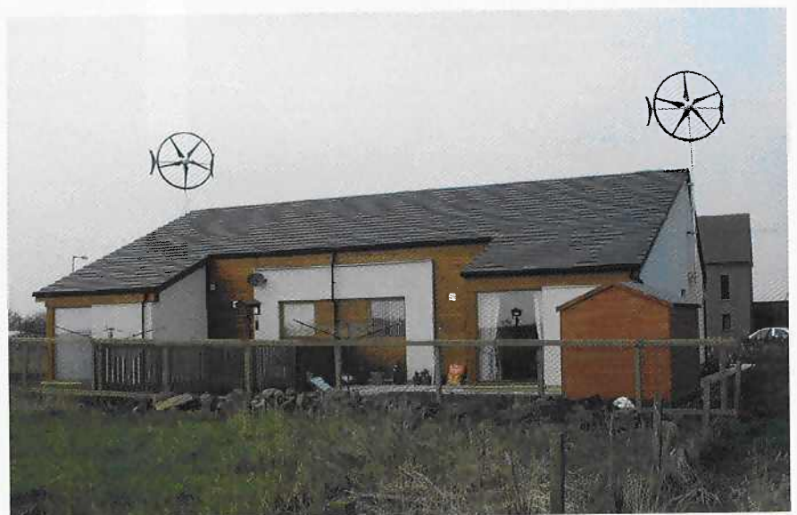
Two turbine configuration on a house. Photo: Berwickshire Housing Association
