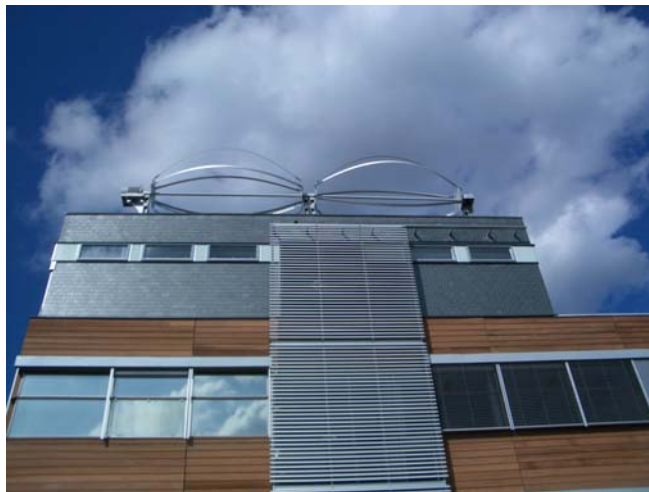
Figure 57: WindWall on the rooftop of the municipal building in Oost Watergrafsmeer, Amsterdam
