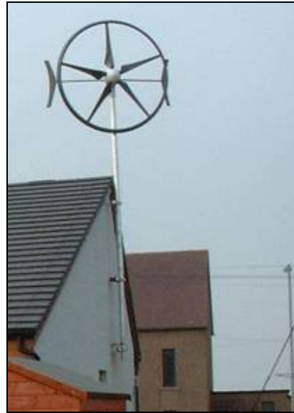
Figure 26. Swift turbine mounting pole (fixed externally)
