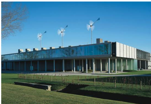
Figure 11: artist impression of urban turbines on the railway building in Den Haag
