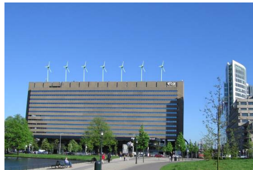
Figure 12: Fortis Montana turbines on the university building in Renson, Belgium
