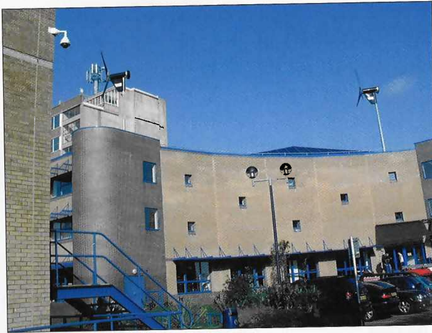
Two rooftop mounted Proven turbines
